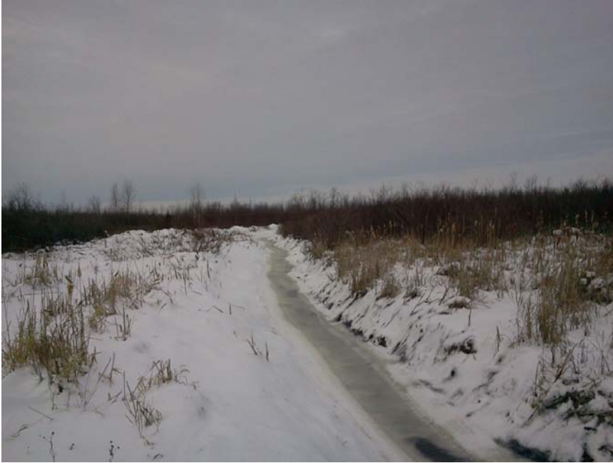
Figure 4.3 Cleaned and excavated drain north of Project Location. (February 2012 - Photo Ref 2)
